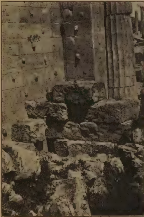
FIG. 20.—Anathyrosis from wall of Propylaea, Athens.
